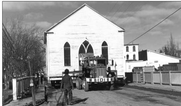
Deconsecrated Baptist Church is transferred over bridge via flatbed.
