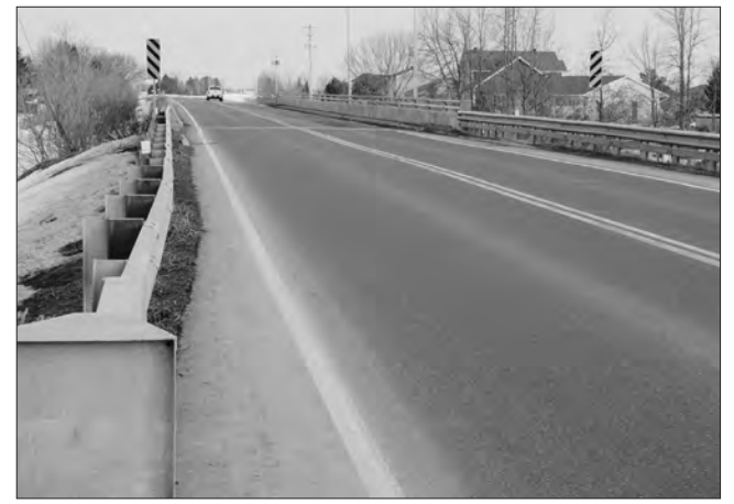
The South Nation bridge, which was built in 1971 will be undergoing a rehabilitation that will require County Road 43 to be closed and all traffic detoured through the Village of Chesterville from May until October.
